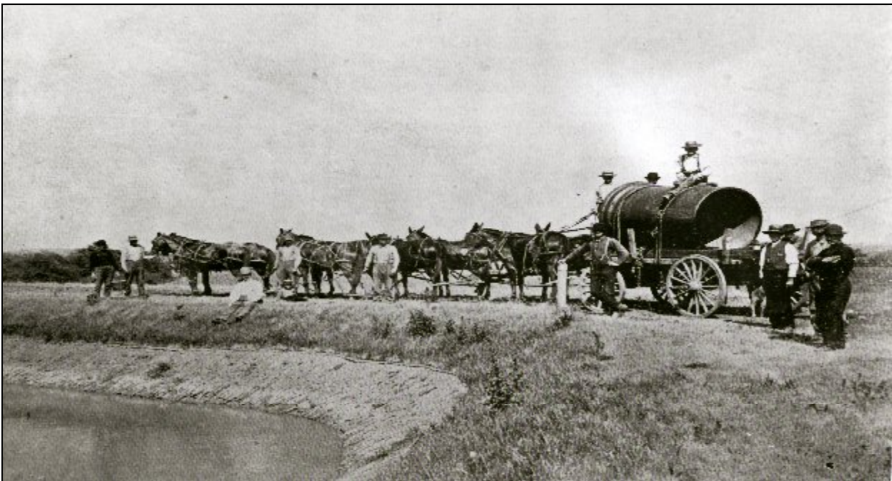
Water Main Construction in St. Joseph, ca. 1894 (Courtesy State Historical Society of Missouri, Columbia)
