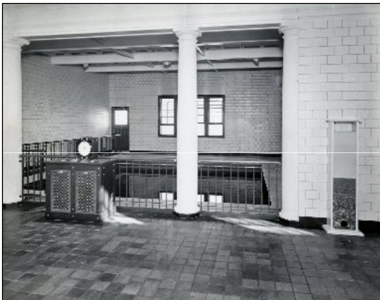
Filter Gallery, Fulbright Plant, Springfield (Courtesy City Utilities of Springfield Archives)
