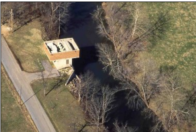
A River Intake (Courtesy City Utilities of Springfield Archives)
