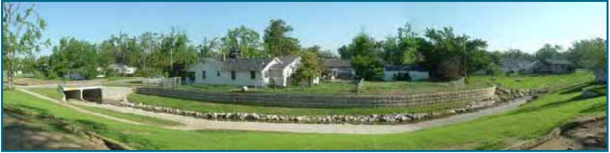
Picture 2. Jordan Creek Daylighting Project (Springfield MS4 Report, 2007). This entire portion was previously in an undersized box culvert. Small fish are now prevalent in the base flow stream, and the trail system is heavily used.
