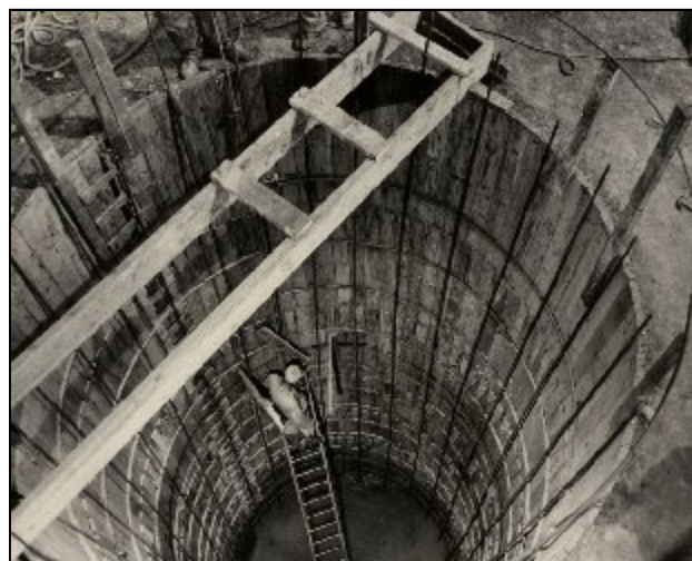
Elevated Water Tank Under Construction (Courtesy City Utilities of Springfield Archives)
